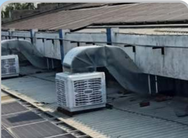
Steel Industries Cooling
